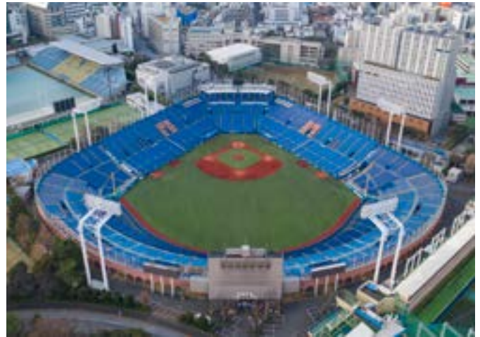
An aerial view of Meiji Jingu Stadium in Tokyo
