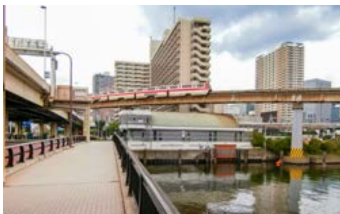
A train on the Tokyo monorail, which began service in September 1964, crosses the Goshiki-hashi (five-color bridge), in Minato ward, Tokyo. The bridge was named for the doomed 1940 Olympics.
