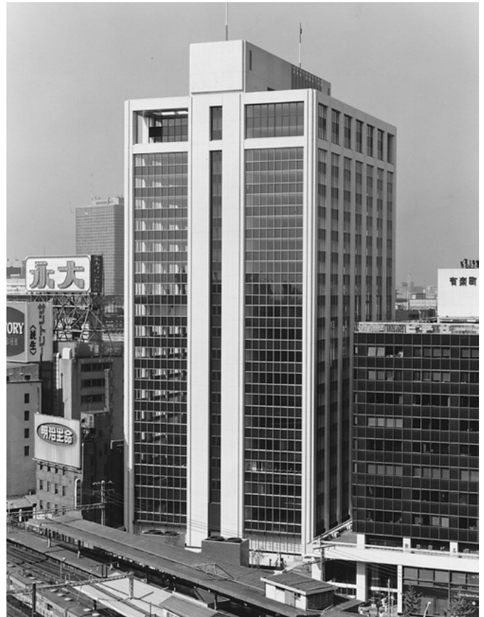
Our fourth club house on the 20th floor of the Yurakucho Denki Building
